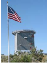
ACC Radar Tower
